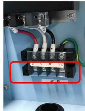
3. Connect the power supply side of the power cable to the power supply.
